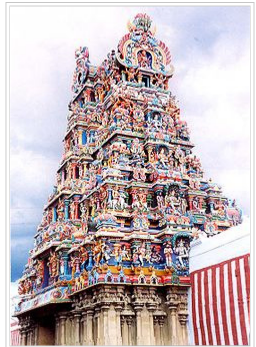
One of the Gopuram of Meenakshi Amman Temple at Madurai
