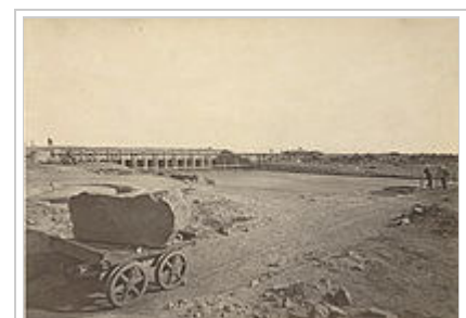
Agra Canal headworks at Okhla barrage, Delhi. 1871.
